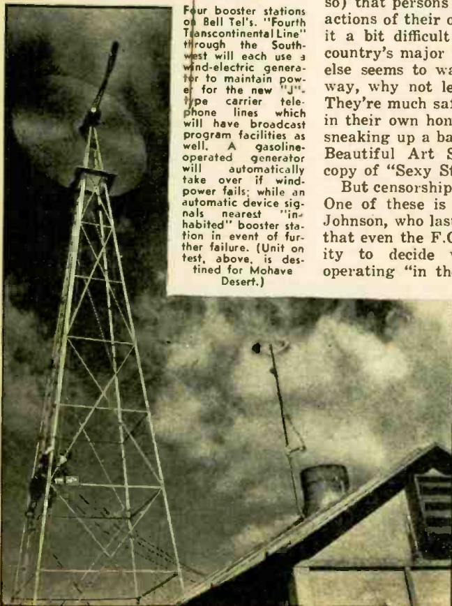
WINDS TO HELP RADIO PROGRAMS. Checking graphed performance of Bell Tel. wind-electric generator, atop Schooley's (N. J.) Mountain.
